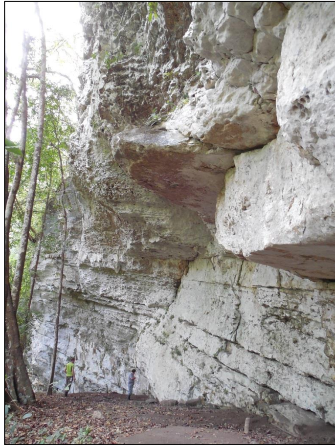
Figure 2.4. Mayahak Cab Pek Rockshelter with Drs. Robinson and Prufer for scale. Note the bedded limestone reflecting geologic unconformities on the rock face. (Photograph by A. Thompson)
